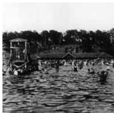
Holzbauten von Ludwig Hoffmann, 1924 Wooden constructions completed in 1924, designed by Ludwig Hoffmann Landesarchiv Berlin
